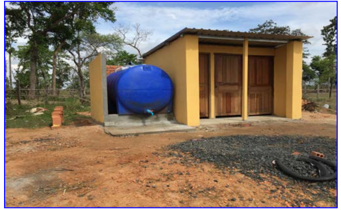
After Toilet Project
