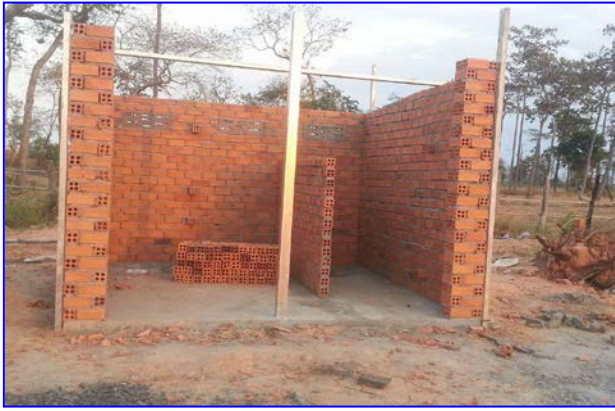
Before Toilet Project
