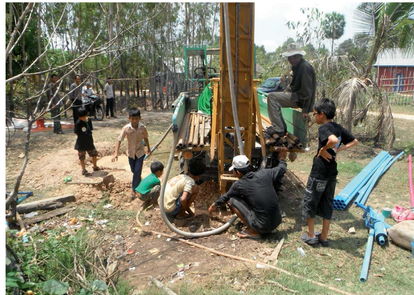
Digging a well
