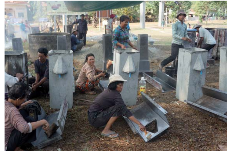
Each family is responsible for constructing their own BioSand Filter
